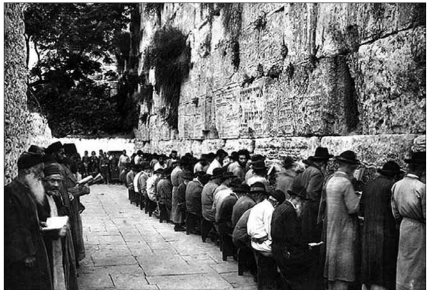
The Western/Al-Buraq Wall, 1929
